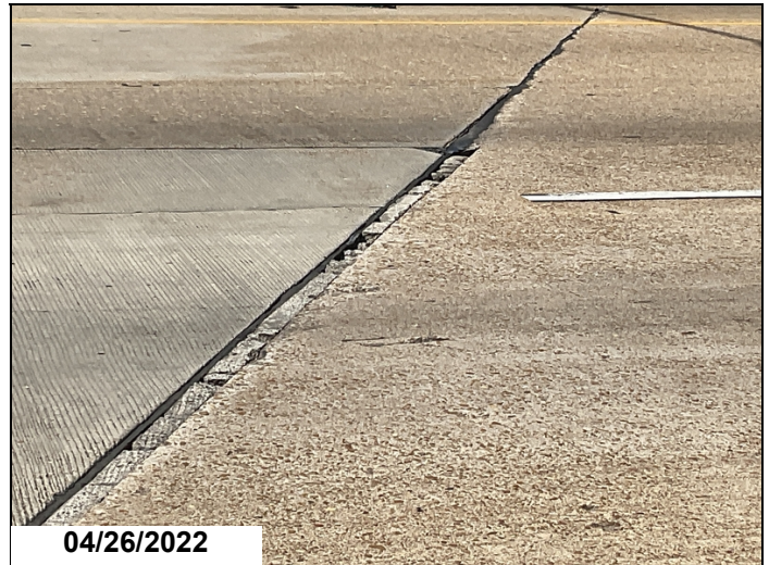
Abutment #2 joint left side adjacent header has twenty feet of cracking and spalling
