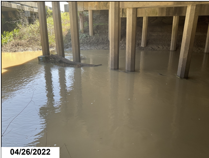
Small drift in channel, bent #3 left side
