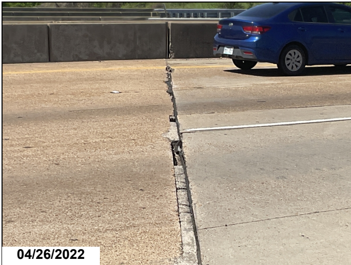
Abutment #1 joint left side adjacent header spalled for six feet
