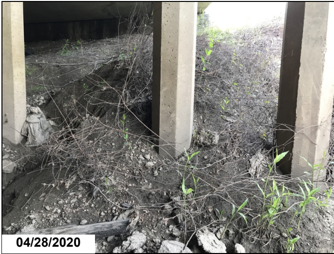
Abutment #1 slope erosion.
