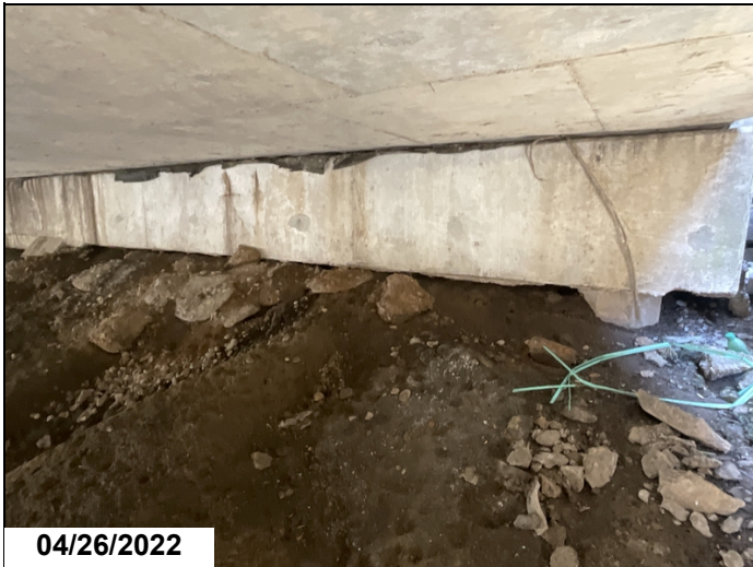
Abutment 2 right end is undermined up to 1' for 15'.
