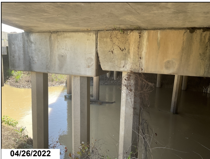
Bent #2 cap back face, left side spalled at construction joint
