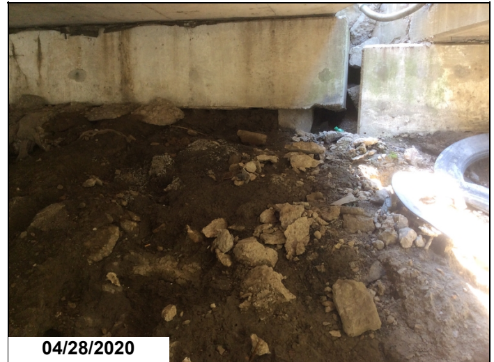
Abutment 2 right end is undermined 1' for 3'.
