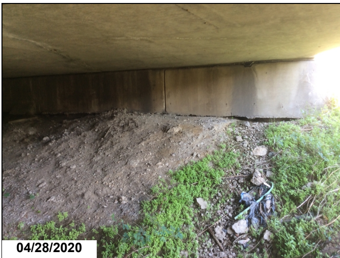
Abutment 1 cap undermined left end.
