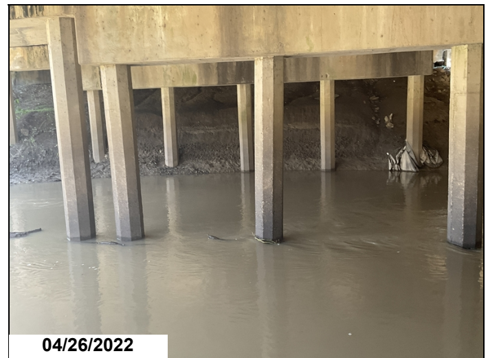
Erosion at bent #4
