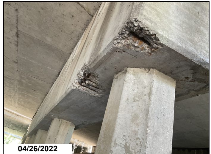
Bent #2 cap ahead, bottom face has two one foot spalls with exposed rebar by pile #5.
